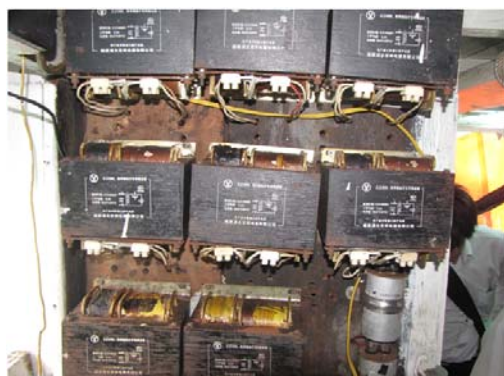
Figure 1 Ballasts of onboard lamps
