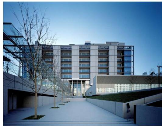
Figure 1 View of Exterior Building Facade
