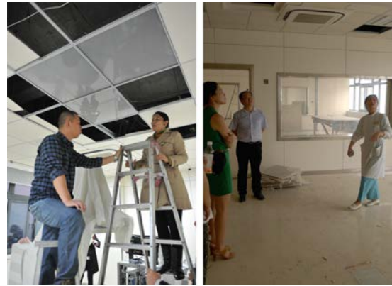
Figure 1 Before lighting renovation
