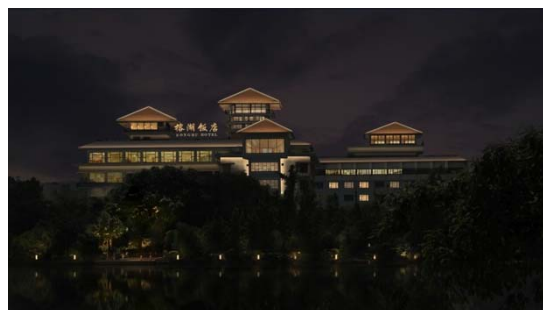
Fig.7 Lighting mode on Ronghu Restaurant
