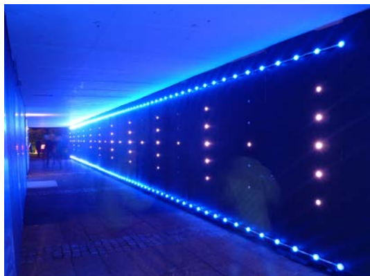
Figure 4 Tunnel lighting installation
